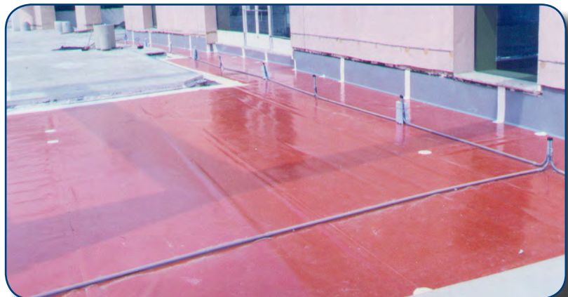
Between Slab Membrane installed over concrete deck
