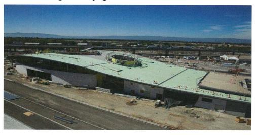
Spanning 10 miles, the BART Silicon Valley Berryessa Extension project is the first phase of construction that includes work on the stations' roof, along with the roof and side screens of the pedestrian overcrossing and installation of skylights in the roof of the station, allowing natural light into both the concourse and the below-ground passenger boarding area.
